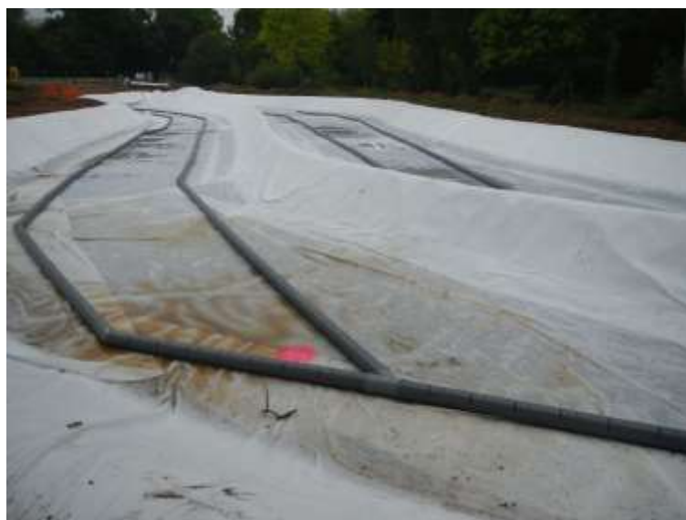
Figure 1. The merging of the two upstream underdrains into a singular section of the same size prompts inquiry regarding how this distinctive setup affects flow distribution throughout the underdrains.
